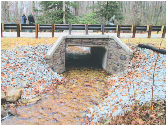
Bottomless culverts are one strategy DCNR has adopted to prepare for increased weather events due to climate change
