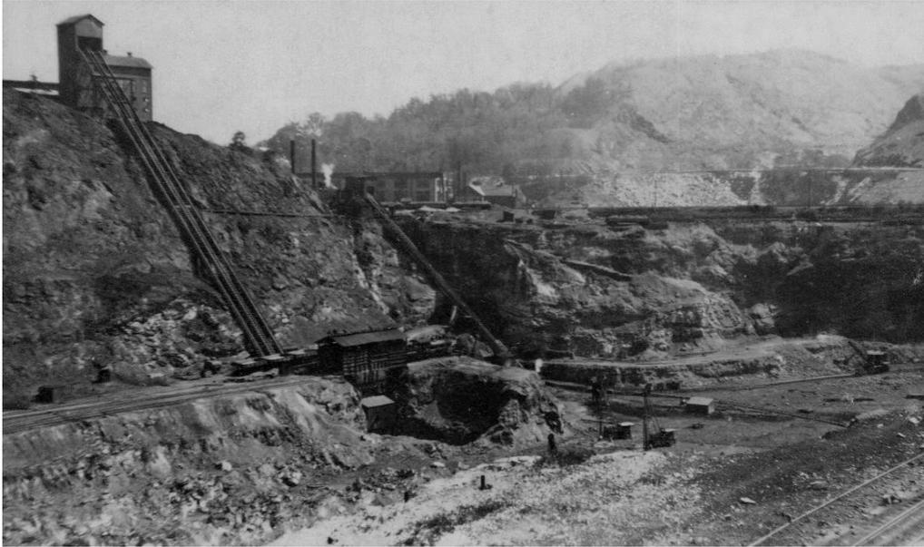
Former State Geologist (from 1919 to 1946) George Ashley took this photograph of the Cornwall ore bank on May 23, 1925 (see the article on [page 3](#)). In 1910, a skip hoisting incline was built, “increasing production by reducing the rail haul” (shown here on the left side of the photograph).
