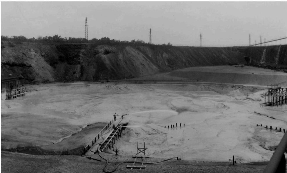
*Figure 4. Removing tailings from the “Old Quarry” for reprocessing at the Lebanon concentrator plant in the 1950s (from the Cornwall Iron Furnace photograph archives).*
