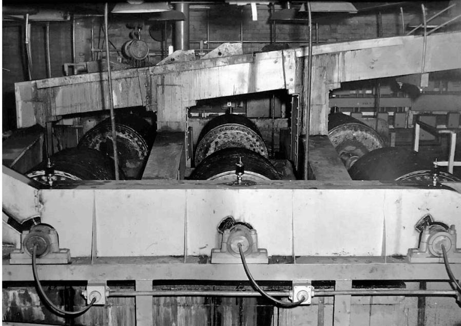
*Figure 3. Six-drum magnetic separators used to separate magnetite ore from the other ore components (from the Cornwall Iron Furnace photograph archives, photograph B-1431).*
