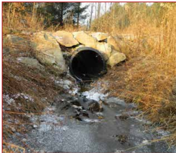
Figure 4.10. Pipe on first order stream perched and too narrow for the natural stream bed. The company has agreed to replace the pipe with an open bottom arch.
