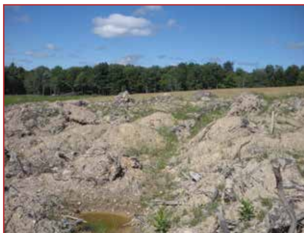
Partial well pad reclamation in Sproul State Forest, following the use of methods similar to ARRI soil dumping (compare to soil ripping photo below).
