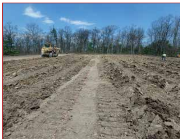
Pad reclamation study site Tiadaghton State Forest, following soil ripping methods: 8" ripping depth on left, compared to 20" ripping on right (compare to ARRI dumping method photo above).
