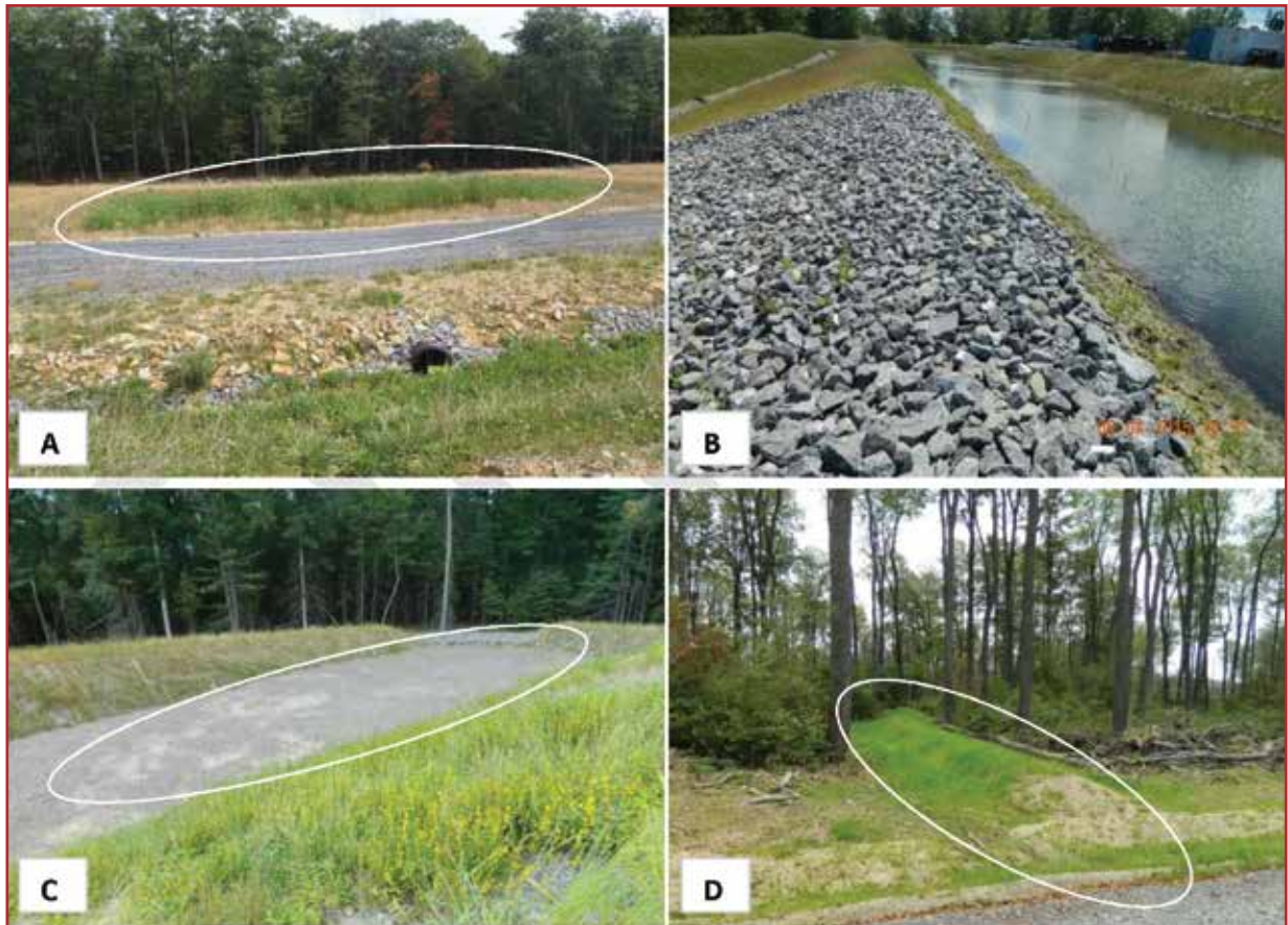
Figure 4.20. Post construction stormwater management practices. A. Water garden, B. Retaining pond with overflow, infiltration trench and basins, C. Infiltration basin, and D. infiltration berm.
