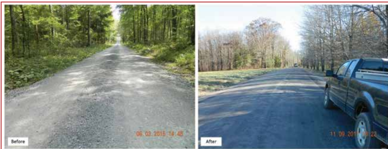
Figure 4.5. Typical high use public road before (left) and after (right) improvement for oil and gas use.
