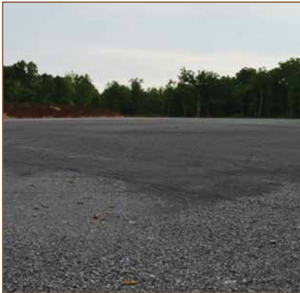
Completed well pad subject to subgrade stabilization.
