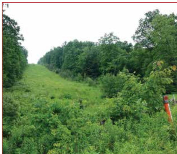
Example of site reclamation on pipeline right-of-way. Note scrub-shrub habitat in temporary workspace on right side of pipeline right-of-way.
