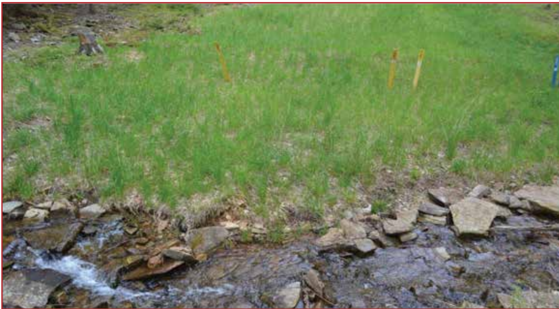
Figure 4.17. Light bank sloughing on the left bank of the right-of-way in the Tiadaghton State Forest.
