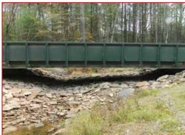
Figure 4.11. Example of bridge on first order stream with clean fill in the stream channel impeding aquatic organism passage. Water passes under the substrate causing disconnected habitat. In clean mountain streams it can take years for the open substrate to fill in.
