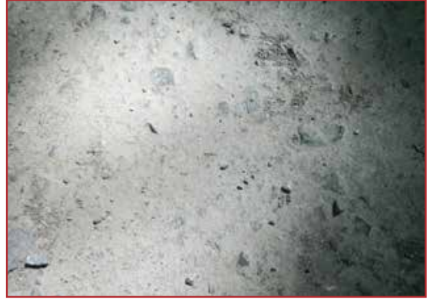
Figure 4.9. Gravel road after application of a petroleum emulsion to control dust, notice the road surface has hardened like pavement.
