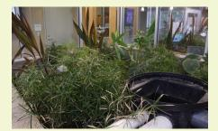
**9. Biological Wastewater Treatment:** A series of indoor and outdoor treatment tanks and constructed wetlands remove waste and clean the water. Treated water is reused for flushing toilets: reducing domestic water use, chemical use, and the amount of wastewater entering Ohiopyle Borough's treatment system.
