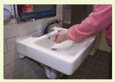
**10. Low Flow Fixtures:** To enhance water conservation, all urinals are waterless and all toilet fixtures, faucets, etc. are of low flow, high performance design.
