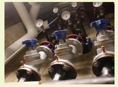
**11. Geothermal:** The building is heated and cooled using earth's stored, thermal underground energy. In winter, the system moves stored heat from the ground into the building. In summer, the system does the reverse. The building's exhaust heat is also recaptured and used to heat incoming air. These processes reduce energy use and dependence on fossil fuels.
