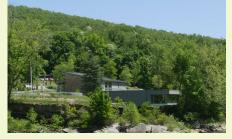
**2. Building Orientation:** The building's orientation maximizes natural light while controlling solar heat gain during occupied hours. The majority of the floor space was intentionally located on the lower level; helping the building blend in with the surroundings.
