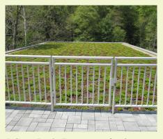
**5. Green Roofs:** Two green roofs reduce stormwater runoff, reduce heat absorption, enhance the insulating value for the interior space, and help the building blend in with surroundings.
