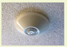
**15. Automated Control Systems:** Automated system controls, like motion sensors and timers, further enhance energy savings and efficiency. Various lighting and heating, ventilation, and air conditioning (HVAC) controls were incorporated to allow for programmable setting adjustments based on levels of activity and occupancy.
