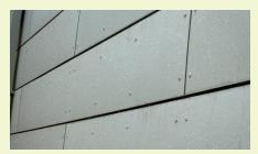
**6. Fiber Cement Rainscreen Installation:** The grey panels on the building exterior shield the building from the elements like traditional siding, but were installed as a rainscreen. An intentional space between the siding and the weather-resistant barrier improves ventilation, minimizing the risk of rot, and reducing direct solar heat gain.
