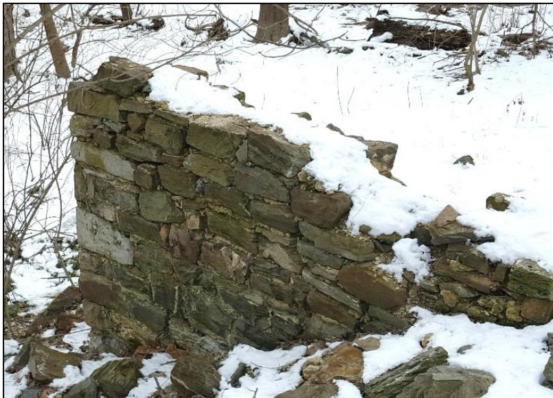
Figure 4. Foundation of smokehouse.
