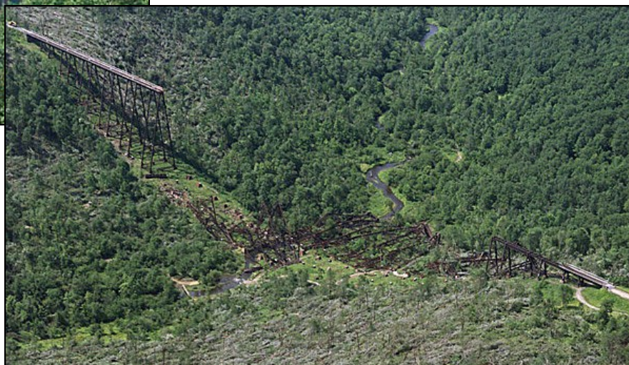
Right: After the tornado, the twisted frame of the viaduct lay on the valley floor (photograph from Pennsylvania Bureau of State Parks).
