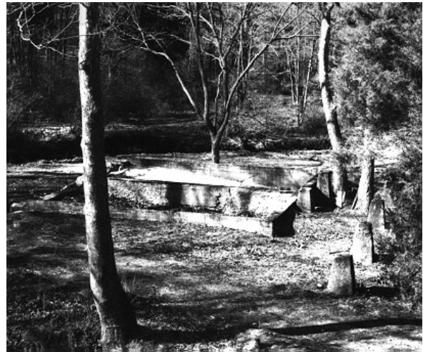
Figure 20. Concrete foundation piers of a mill constructed in NCP during World War I for the recovery of placer chromite.
