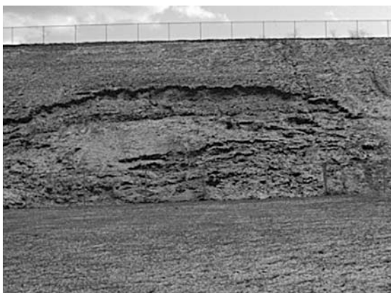
Figure 13. Small slump in the cut portion of a recent cut-and-fill slope. The slumped material is a thick claystone between layers of stronger rock.
