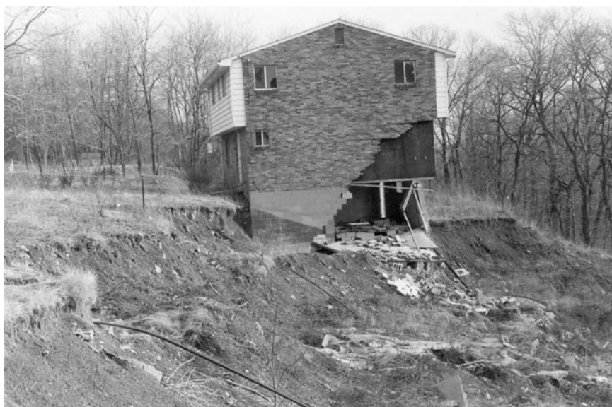
Figure 22. A new home that was severely damaged, and eventually totally destroyed, by slope failure. The remains of the home (since demolished) are at the head of an active slide developed in fill material placed on top of old landslide materials. Photograph by J. L. Craft.
