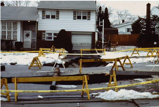
Figure 18. Sudden collapse of a city street attributed to a water-line break in the karst area of Northampton County.
