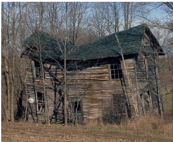
Figure 1. The slow removal of support for this abandoned Pennsylvania farmhouse has caused the roof and side-walls to tilt and sag.
