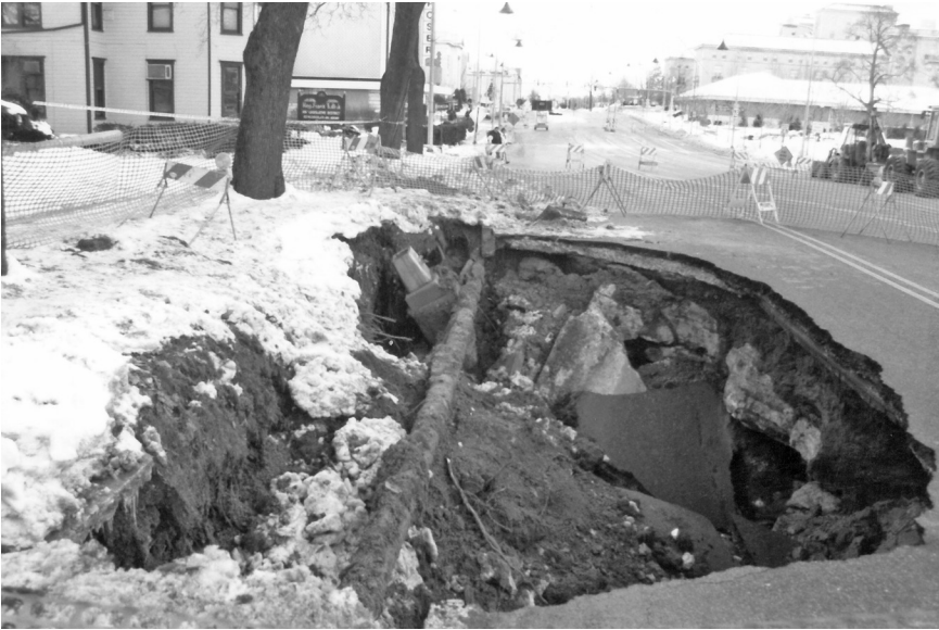
Figure 13. This sinkhole in Dauphin County has exposed a utility pipeline.
