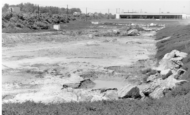
Figure 17. Sinkholes in a storm-water retention basin along U.S. Route 22 in Lehigh County.
