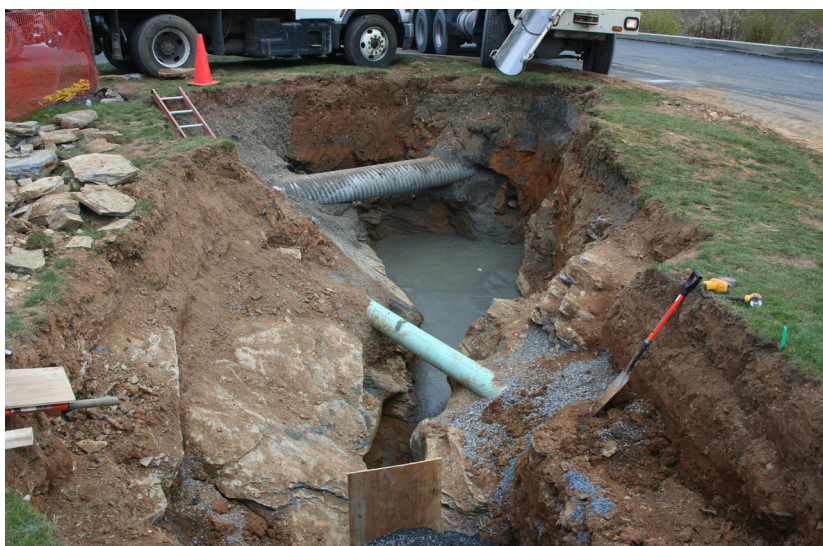
Figure 19. Sinkholes often affect utility lines. In this instance, the void between the exposed bedrock has been filled with concrete to provide a stable base for additional backfill materials and for the overlying utility pipelines.
