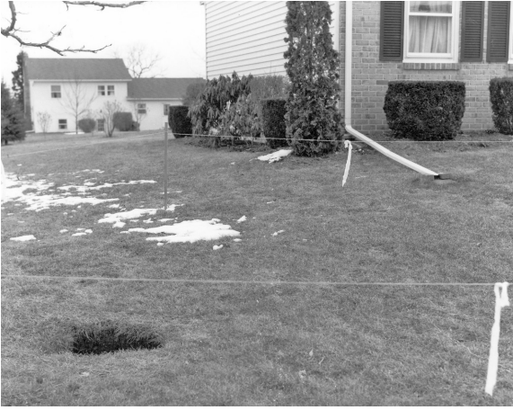
Figure 16. A sinkhole resulting from water discharging from a storm gutter. Sinkhole formation can be attributed to storm-water runoff throughout central and eastern Pennsylvania.
