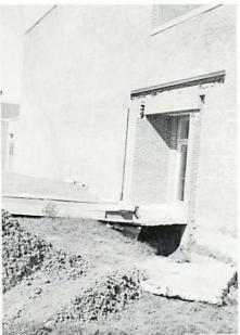
Figure 2. Sinkhole developing beneath entrance to school causing collapse of ground below entrance. (Photo courtesy of J. P. Wilshusen.)
