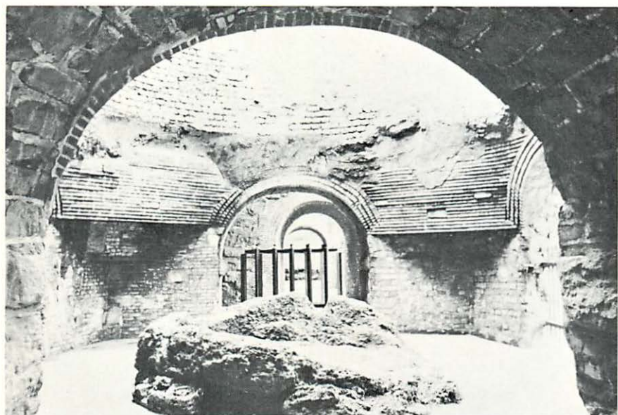
Fig. 2. Large mass of slag at the base of one of the restored furnaces.
