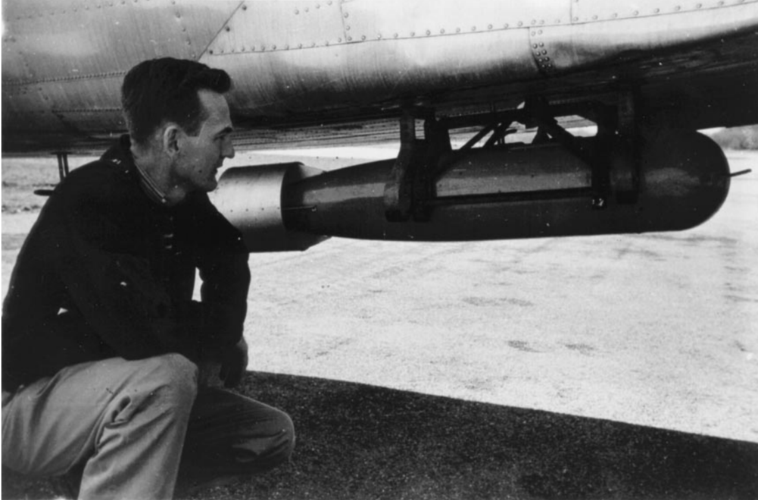
Probably in the 1960s, staff geologist Richard Conlin examined a magnetometer that was mounted on an airplane to survey magnetic anomalies.
