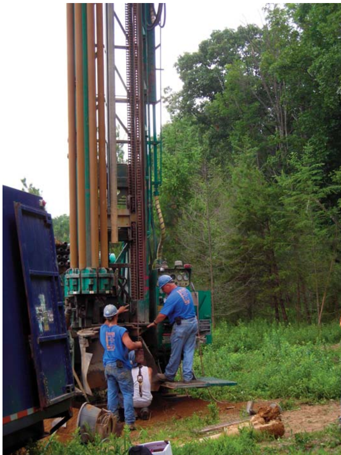
Figure 7. The drilling team (Holt Drilling Co.), preparing to add the 15-inch diameter drill. The top 20 feet of overburden was drilled at this diameter to set temporary surface casing. Photograph by Aaron Bierly.
