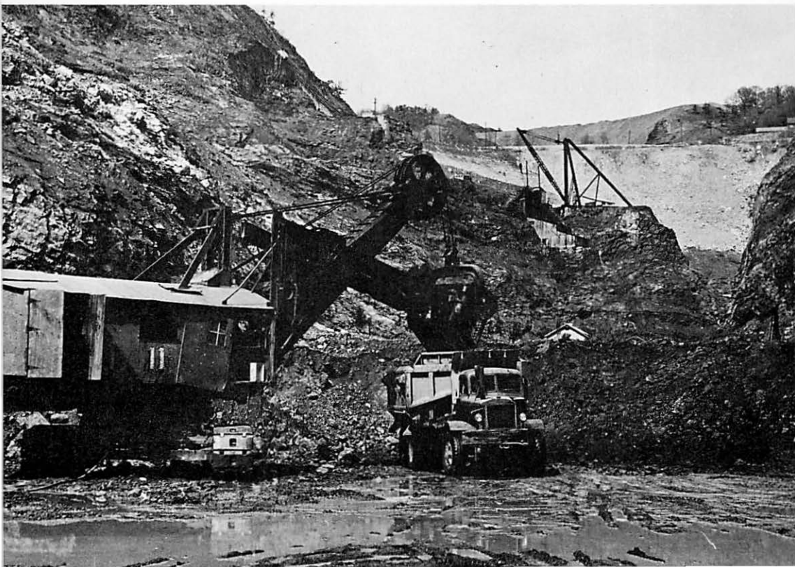
View of main open pit mine, 1952. Ore shows as black zone at base of left wall, with light-colored overlying limestone. Right wall of pit is south-dipping diabase.
