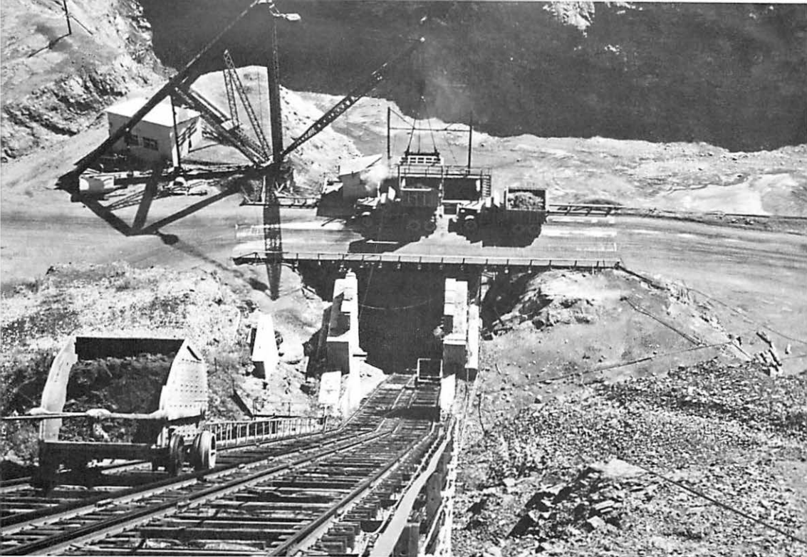
Skip bringing up ore on inclined shaft of No. 3 mine, 1952.
