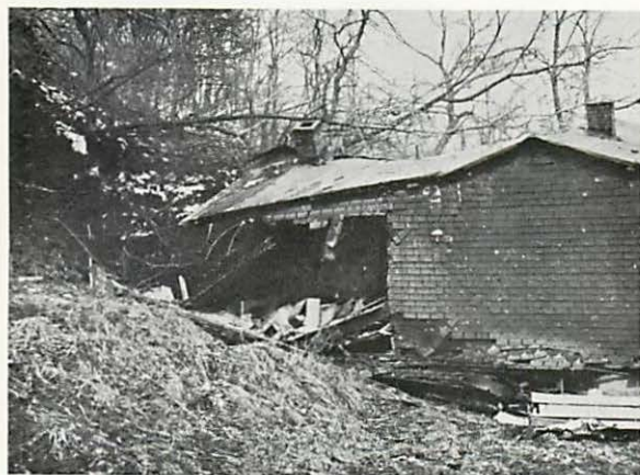
Home being crushed by toe of slide, along Route 28 near Millvale.
