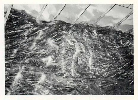
Figure 3. Shear zone in the Martinsburg Formation exposed in the new Lehigh Tunnel on January 24, 1990, believed to be the floor thrust of a duplex in the Shawangunk and Bloomsburg Formations. Welded wire fabric and spilling pipes at the top are part of the "shotcrete" canopy used to reinforce the tunnel crown and protect the tunnel opening.
