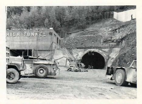
Figure 5. North portal of the second Lehigh Tunnel excavated in the Bloomsburg Formation. Bedding is overturned and nearly recumbent. Note the elliptical shape of the tunnel bore, a diagnostic feature of the New Austrian Tunneling Method.
