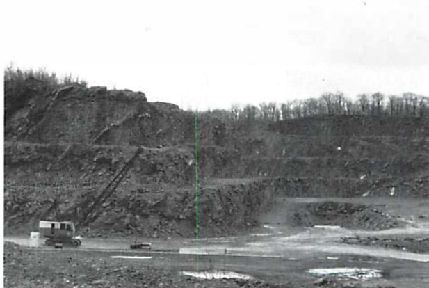
Figure 1. Southwest-looking view of the West Ridge quarry of GAF Corporation, showing the five levels of bench development. Faint southeast-dipping cleavage is visible in the near faces.
