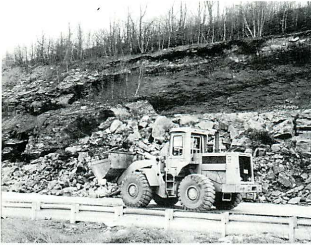
Figure 3. View of the northeast end of the rock-slide, showing the large intact block adjacent to the side scarp. Note the subvertical head scarp.
