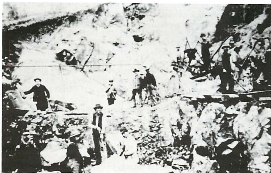
Figure 1. Photograph of the J. E. Baker Company's now-abandoned Billmeyer Quarry near the turn of the century showing the process of drilling dolomite.
