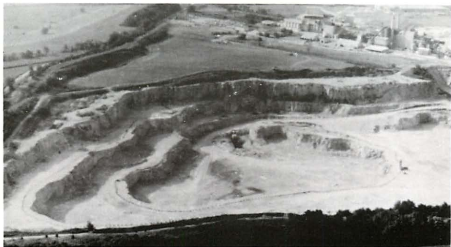
Figure 2. A southwest-looking view of the J. E. Baker Company's active quarry and plant. Quarry benches are about 50 feet in height. A sense of scale can be achieved by comparing the size of the production drill located on the 3rd level, bottom right of photograph.
