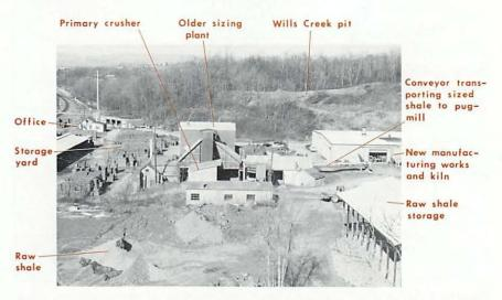
Figure 2. View of Watsontown Brick Company operation from the ridge south of the plant looking north.
