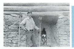
Fig. 5 Samuel W. Berkheiser, Jr. tending the initial 3-5-hr. burn in the firebox. Notice long pole to the left with forked hooks used to extract the lump lime through the keyhole, which is clearly visible at rear of work chamber.
