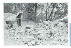
Fig. 3 Arthur L. Long using stonefork to load sized limestone. Notice 16-lb. sledge in foreground.
