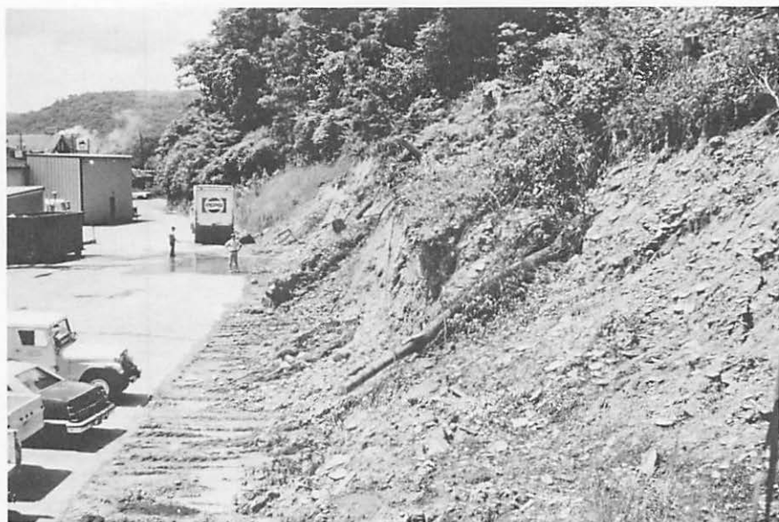
Fig. 2 Base of colluvial slide. Parking lot previously had been covered by soil and rock debris.
