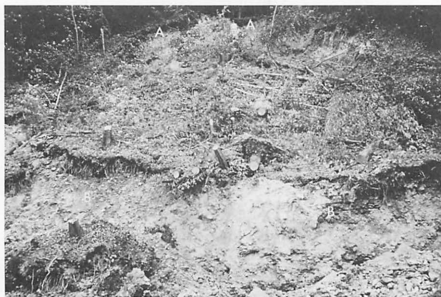
Fig. 3 View of slide looking upslope from parking lot. Note scale in front of head (A). B is foot of slide.
