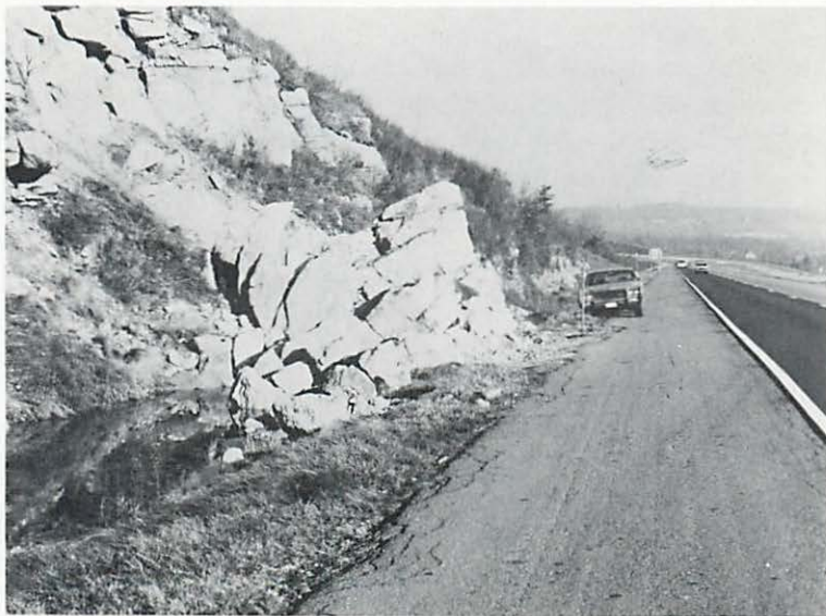
Figure 1. Rockfall from a road cut in central Pennsylvania.
