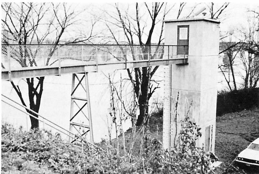
Susquehanna River monitoring and gaging station at Harrisburg: Historic flood marks are marked along right edge of scale on building; flood stages recorded for 1975, 1972, 1936, 1894, 1889, and 1784.
