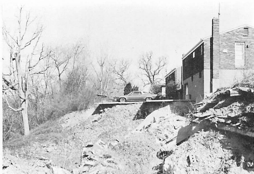
Figure 4. Upper portion of a large complex slope failure in western Pennsylvania.
