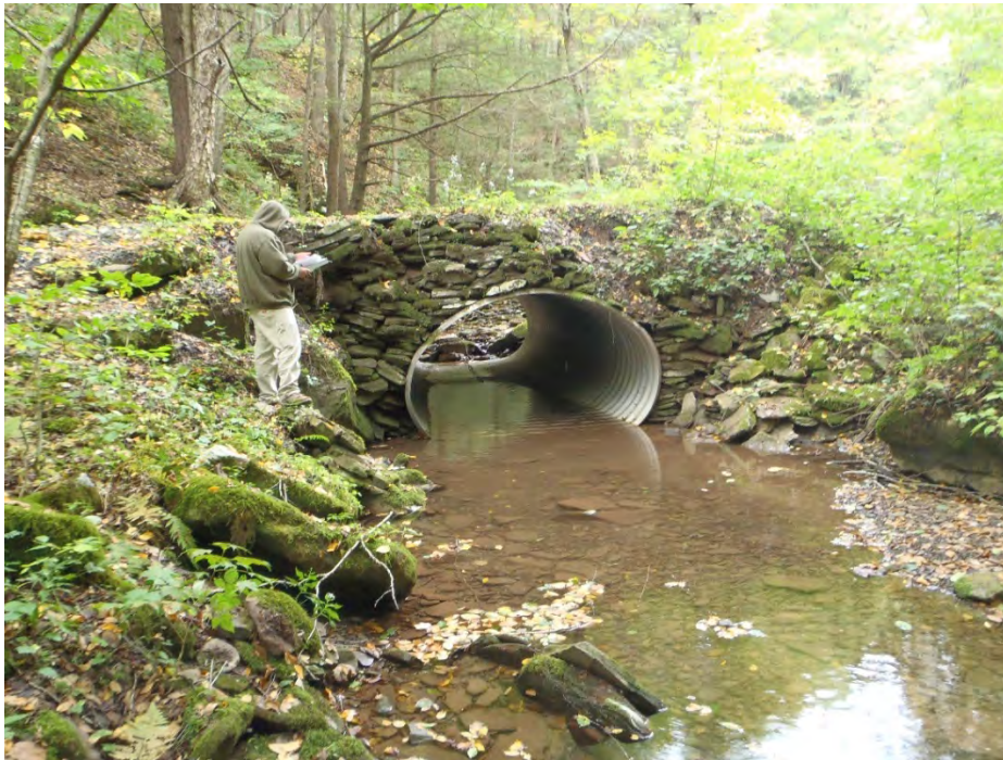
Culvert being assessed for Aquatic Organism Passage
