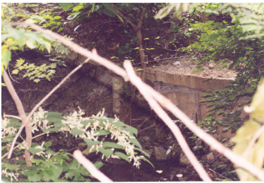
5. Broken concrete bulkhead Action/BMP: Have the township engineer assess the problem and develop solution.
