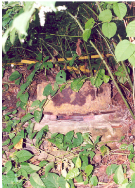
6. Broken/breached concrete collar of sanitary sewer Action/BMP: Have the township engineer assess the problem and develop solution
