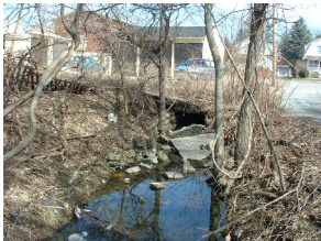
1. The culvert outlet at Tyson and Mount Carmel Avenues is small (approx. 2' by 3') and is blocked by cement slabs. Action/BMP : Have Cheltenham Township remove concrete and conduct routine monitorings in the future.
