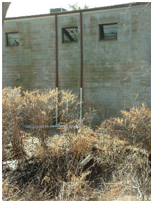
5. The businesses on Glenside Avenue have their stormwater downspouts draining directly into the creek via PVC piping along the right bank. Action/BMP : Encourage businesses to use rain barrels to slow volume of water entering the Tookany Creek, and also to reuse on-site.
