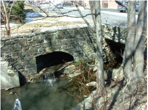
7. The creek makes a 90 degree turn under Glenside Avenue, becomes channeled and flows between and behind homes, before discharging into Grove Park. Culvert headwall shows finely skilled stonework of local masons that can be seen throughout the area. Action/BMP : None necessary.
