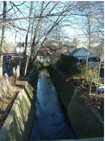
11. The unknown tributary flows under Harrison Ave. becomes channelized again, flows beside and behind homes where it makes a 90 degree turn then meets the main stem of the Tookany behind the old Boston Market on Easton Road. Action/BMP : Consider biotechnical streambank stabilization, regrading banks and replanting with native vegetation.
